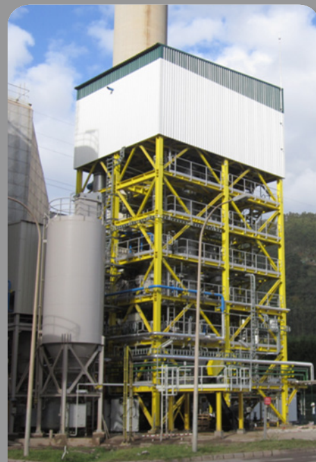
1.7MW Calcium Looping test facility at the La Pereda power plant in Spain where continuous testing has been undertaken over 1000's of hours at this scale. The next step is to scale the process up to the 20MW scale. Image courtesy of Carlos Abanades, CSIC.
